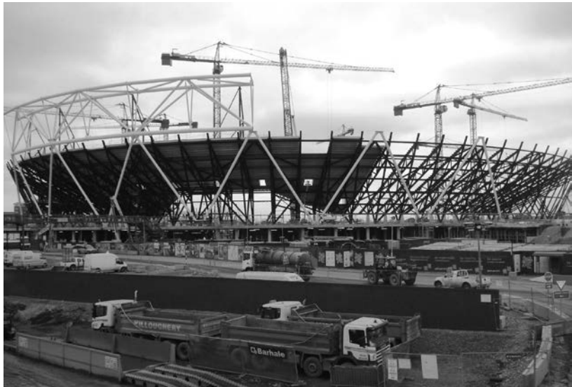
Plate 10: Logistics of the London Olympics: Building the Stadium. Picture: Graham Miller
